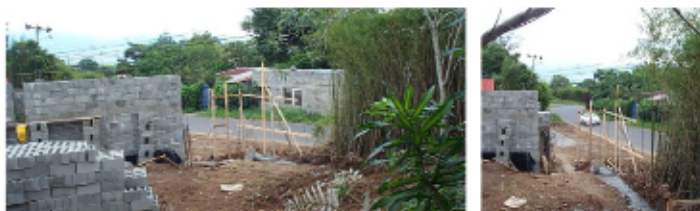
Backyard boundary wall New construction (May 2006)
