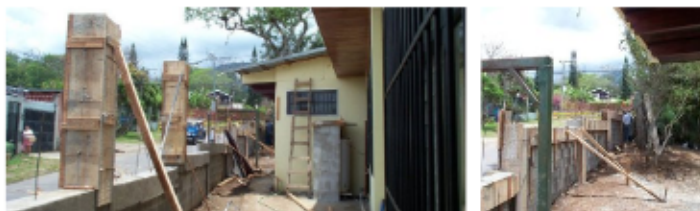
Calle 120 boundary wall New construction (May 2004)
