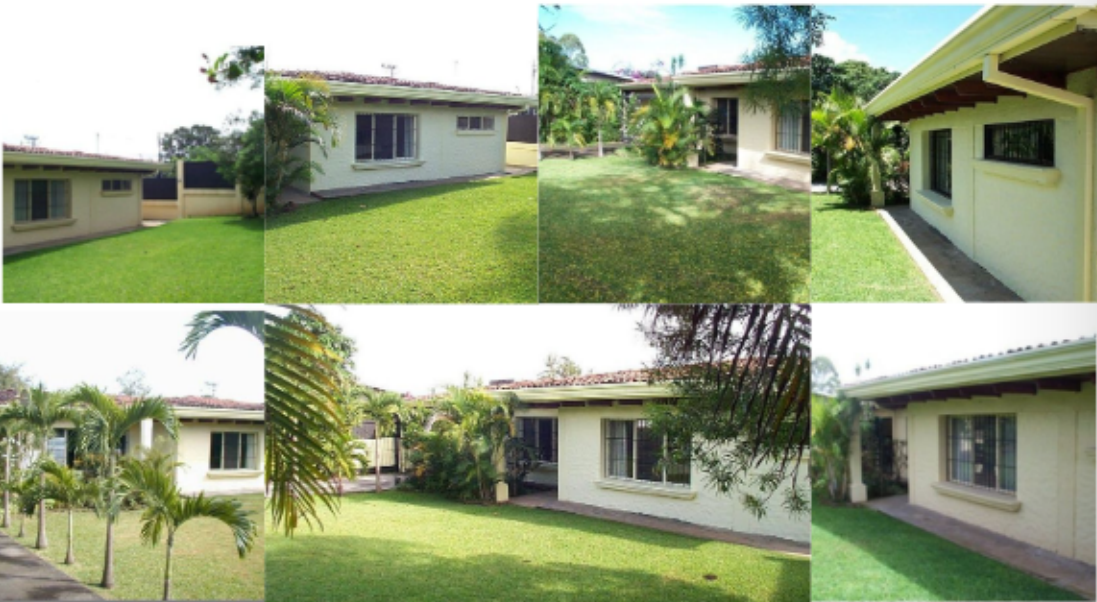
Front of house Renovation & new construction Master bedroom terrace room added
